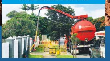
Vacuum excavation uses high-pressure water jets to break up solid ground, whether it's sand or clay, rocks or soil and simultaneously vacuums the debris away, into a holding tank, for disposal after a job is completed. This is a non-invasive, cost effective and accurate way to visually locate underground utilities prior to excavation and reduces the risk associated with damaging these assets.
